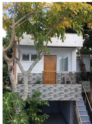
Figure 2. Façade of Disaster Shelter Facing West
