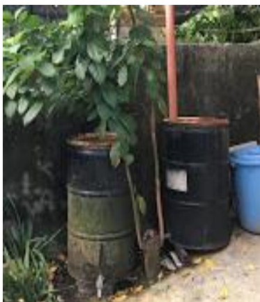
Figure 6. Simple Rainwater Harvester
